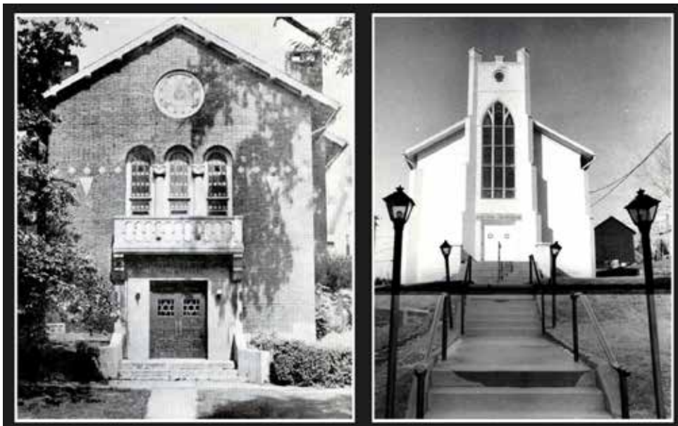
At left is B'nai Israel of Auburn, New York, which was located at 18 Seminary Avenue. The building was demolished in 1974 to make way for a new roadway funded as part of a federal urban renewal project. At right is the former Congregation B'nai Israel of Lancaster, Ohio, around 1990. While the synagogue disbanded in 1993, the building still stands and is now an Airbnb. (Austin Reid; Fairfield County Heritage Association)
