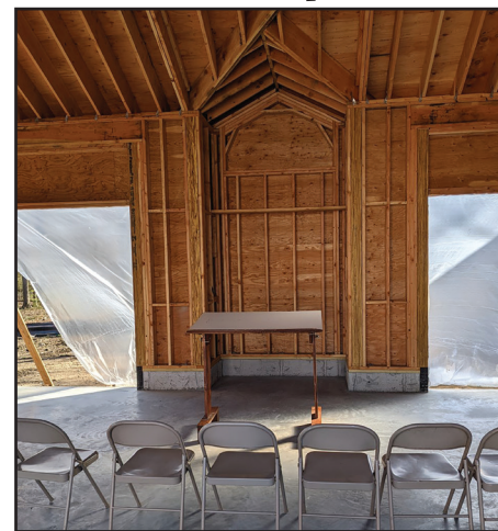
The Chabad House under construction.
