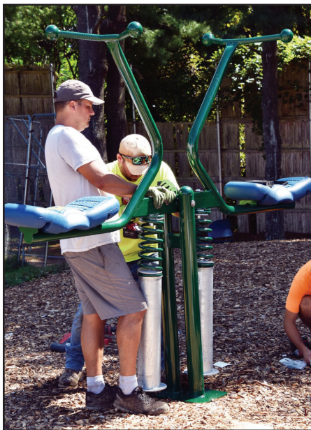
Workers install the new equipment in the BCHA playground area. (ALL PHOTO CREDIT: PAUL SILVERFARB)
