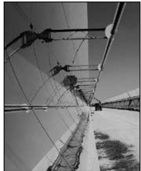
A machine cleaning the parabolic mirrors at the Ashalim Solar Thermal Power Station. (Photo courtesy of the Ashalim Solar Thermal Power Station)
