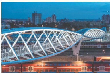
Beersheva High-Tech Park Bridge
