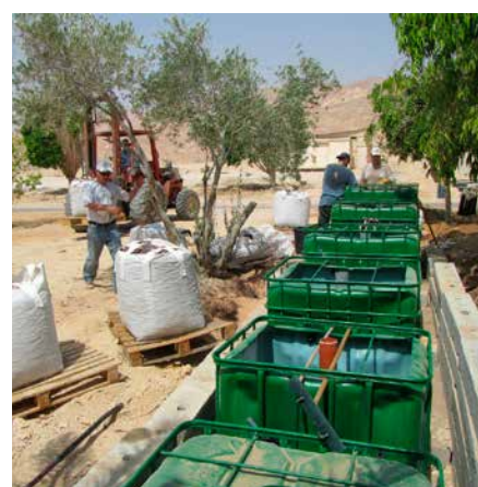
The major components of a greywater treatment and reuse system being installed on the Arava Institute campus to serve some of the dormitories.
