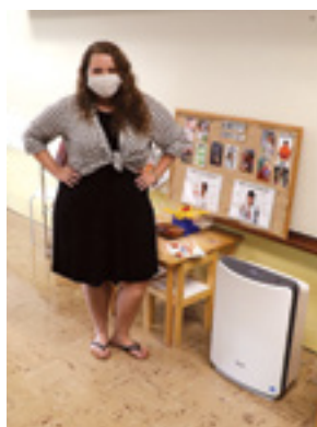
ECDP teacher Rebecca Wojtanowski stands next to one of the new air scrubbers (on the floor) installed in every ECDP classroom.
