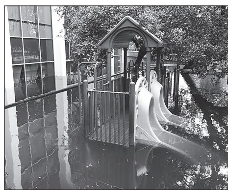
Hurricane Harvey flood damage at the Evelyn Rubenstein Jewish Community Center of Houston. (Photo courtesy of JNS)
