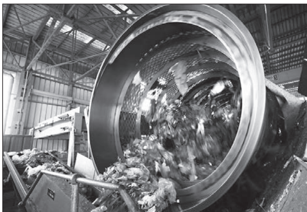
Solid waste treatment facility “Arrow Ecology” at the foot of the Hiriya landfill near Tel Aviv (Photo by Chen Leopold/Flash90)
