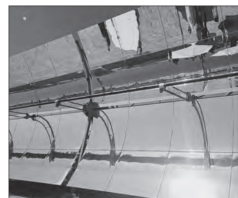
At right: A close-up of one of the parabolic mirrors used at the Ashalim Solar Thermal Power Station. (Photo courtesy of the Ashalim Solar Thermal Power Station)
