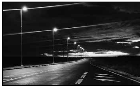
Newly paved street with lights
