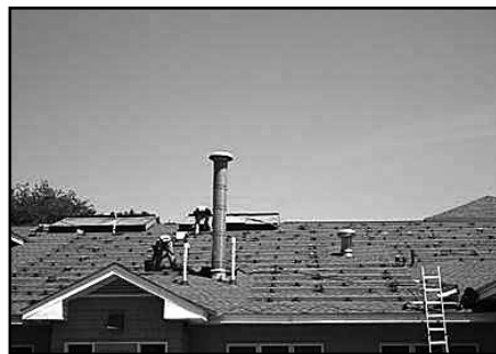
Workers install solar panels on Temple Beth Abraham's roof.
