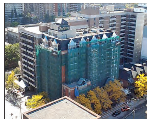
Radisson Hotel – Queen Street
