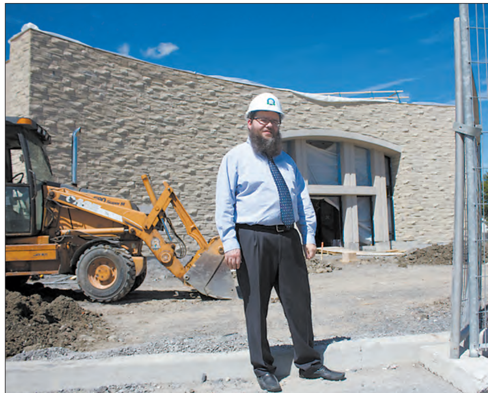
Rabbi Menachem Mendel Blum oversees construction at the site of the new Ottawa Torah Centre Chabad facility slated to open September 15.
