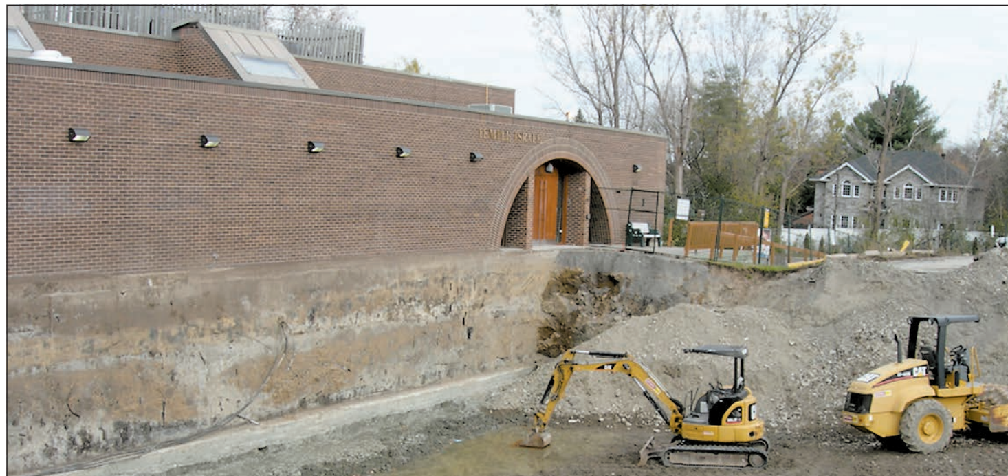
This photo taken November 5 shows the extent of the work taking place beside Temple Israel's front door.
