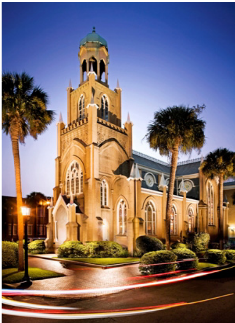
Image by Attic Fire Photography
