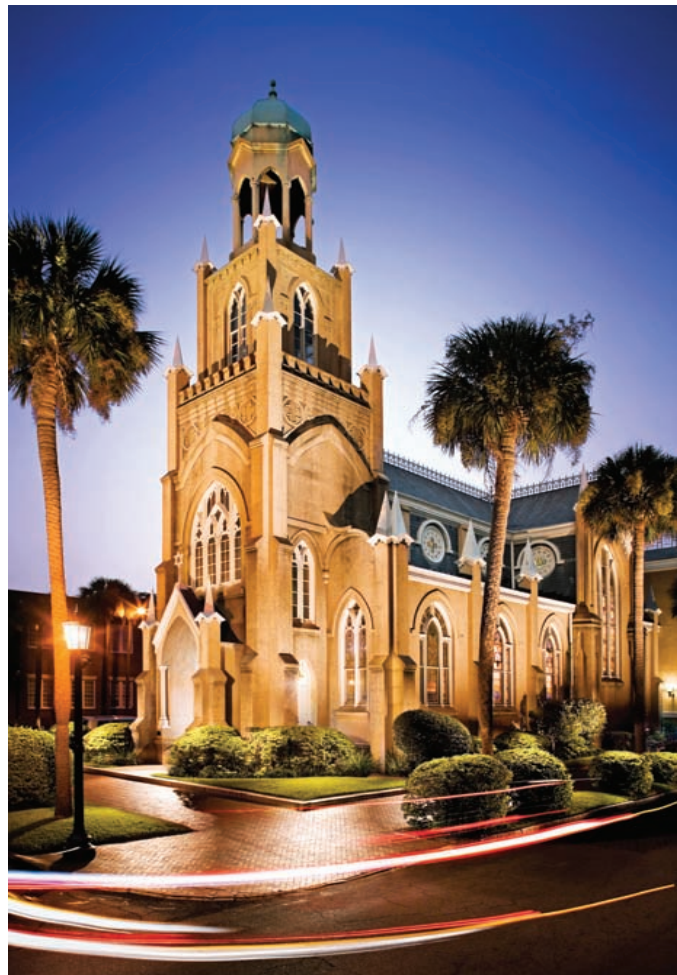
Image by Attic Fire Photography
