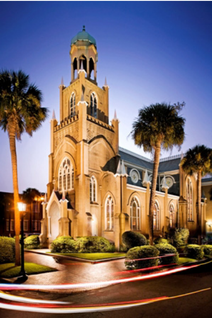
Image by Attic Fire Photography
