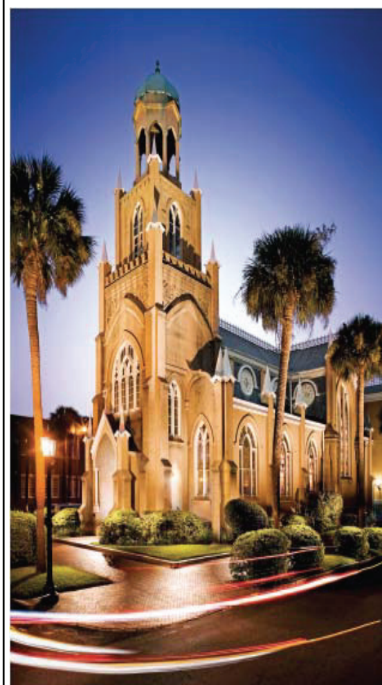
Image by Attic Fire Photography
