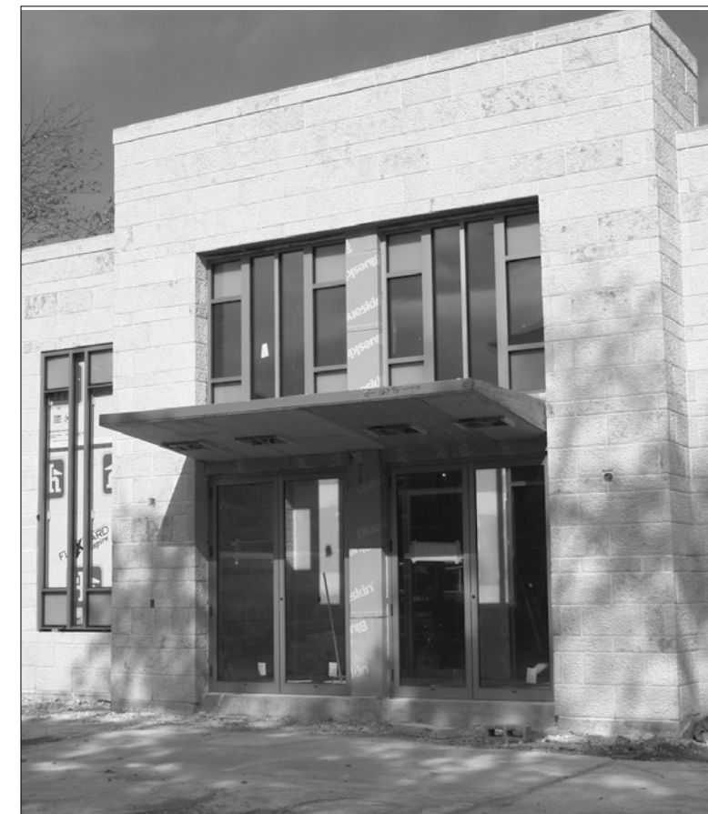
The new shul entrance made of Jerusalem stone on Cottage Avenue.
